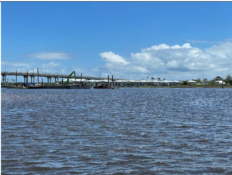
Photo 6: Typical view of offloading point for the smaller barges.
