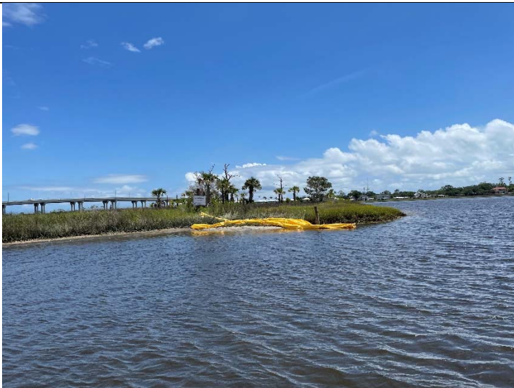
Photo 4: Typical turbidity barrier and manatee signs
