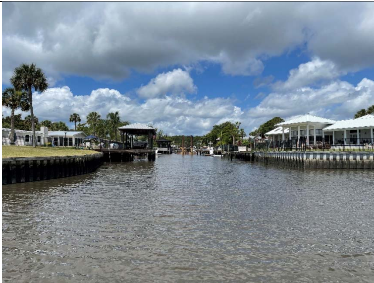
Photo 1: Barge actively dredging in Baseline 6 IOP District.
