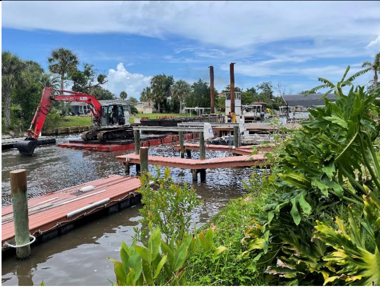
Photo 1: Typical View of Baseline 2, 20' Wide Barge being pushed to off-load.
