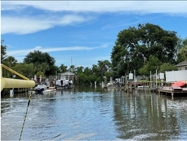
Photo 5: View towards two docks at Station 29+00 in Baseline 2. Docks were measured at the time of the inspection to be approximately 23 feet apart.
