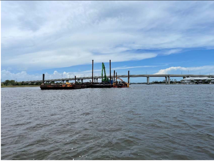
Photo 3: View of 26' Thruster Barge being off-loaded.
