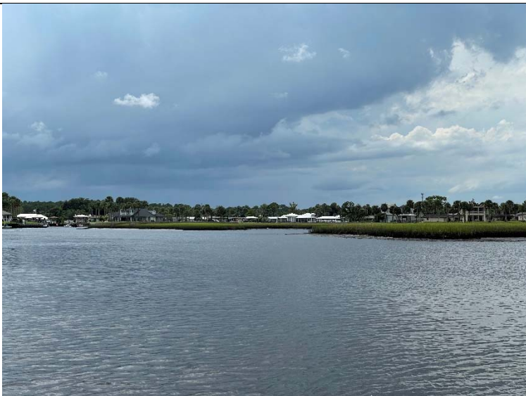
Photo 2: View of Thruster Barge (in the distance) heading back into Baseline 1 to continue re-work of high spots previously identified.
