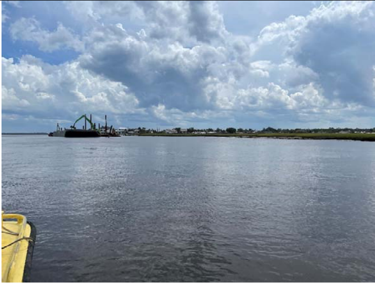
Photo 3: View of 20' Push Barge being off-loaded.
