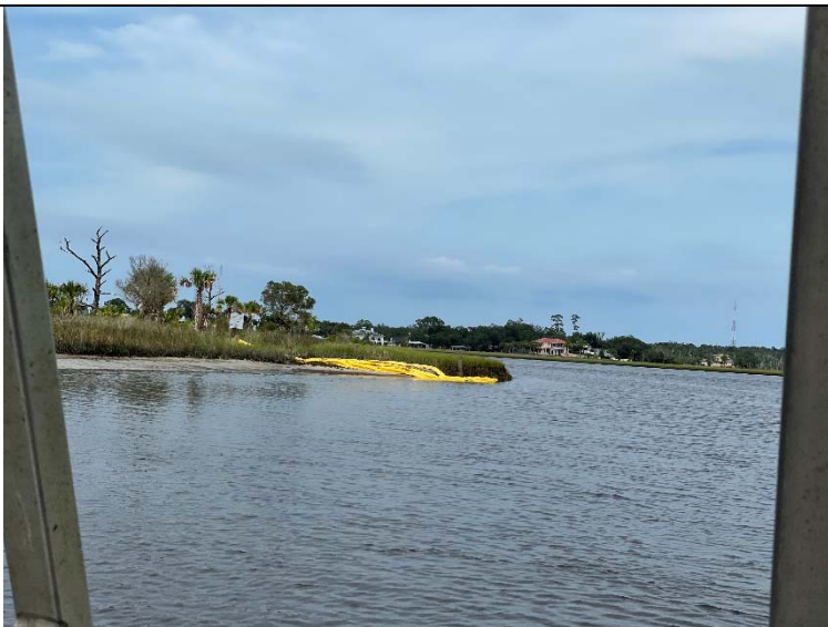
Photo 4: Typical view of turbidity barrier and manatee signs.
