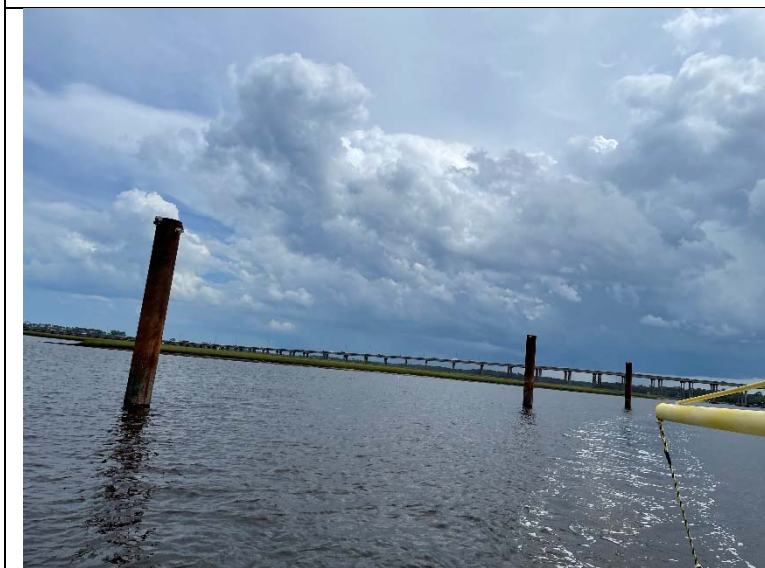
Photo 6: Future location of ~50' Wide x 100' Long hopper barge.
